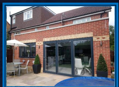
Rear extension in Redhill
