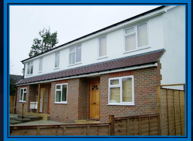
New-build homes in Reigate
